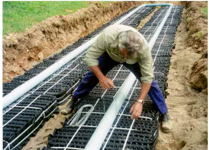
Contractors find geotextile sand filter systems from Eljen Corp. easy to install. Only rough-cut surfaces filled with 6 inches of sand are required.
