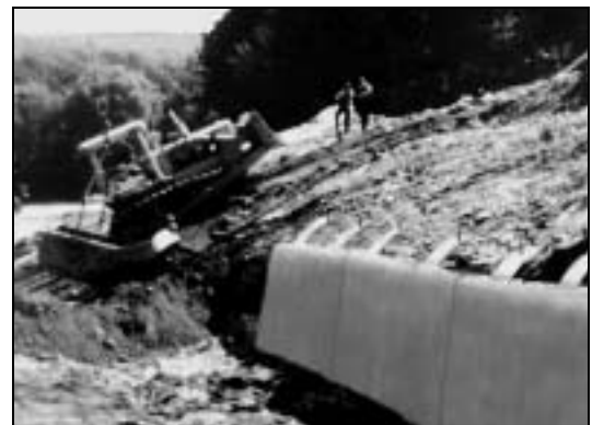
Steps 2 Through 4—Installing and Backfilling the PDS
