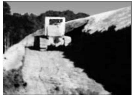
Step 1—A berm is cut
