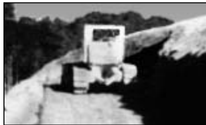
Often, only one bulldozer is all that is required.
