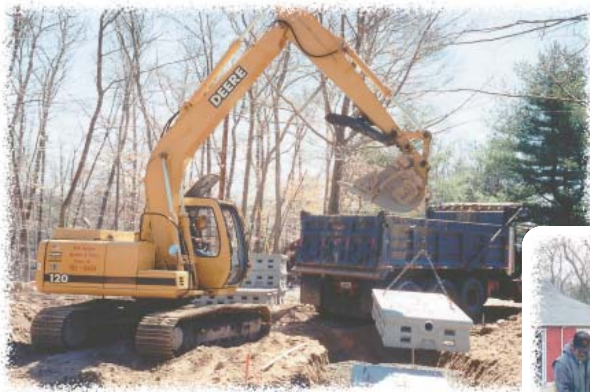
Above, a Superior Septic technician places galleys on top of crushed stone during a septic system installation. At the right, technician Dave Boisclair pumps out a cesspool.
